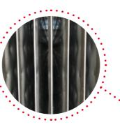
• The flexible connections/ hoses to the plates allow thermal expansion; they make easier also maintenance activities and the eventual replacement of individual plates. The manifold construction is anyway done to avoid the possibility of ambient air intake in the tower;
